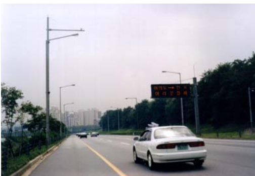
Real-time traffic information collected with Autoscope is relayed to motorists using variable message signs
