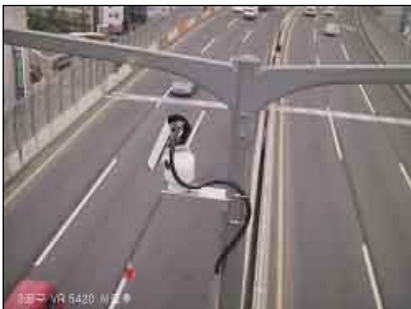
An Autoscope Image Sensor (AIS) on pan/tilt mechanism being used for area surveillance on the Olympic Highway in Seoul, Korea and the AIS being used to collect real-time traffic data for Automatic Incident Detection
